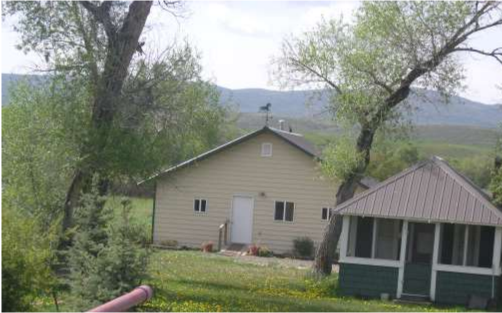
New Bath House - just behind cabins Multi-Stall & Shower Facility
